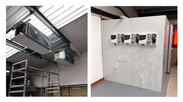
The new system will be used to enhance our one day R744 (C15) course which covers the basics of R744, safe handling and introduces transcritical and booster technology. We will use it to demonstrate transcritical operation and for practical exercises.
