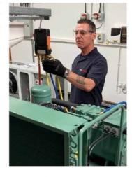
refrigerant is pumped down to the condensing unit and liquid line.
