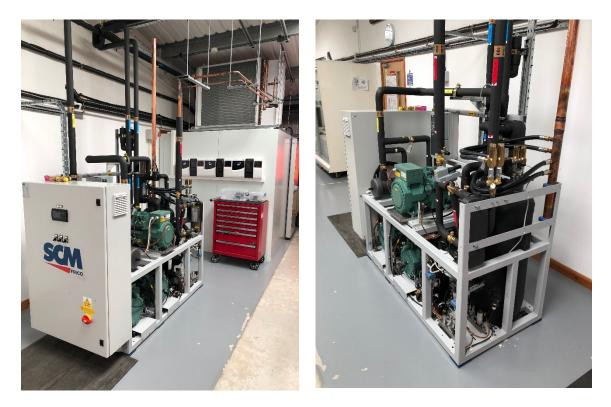
The plant installation follows a period of significant investment in updating the R744 equipment used for training started in February 2018 that saw the decommissioning and scrapping of our first subcritical cascade system installation from 2009.
