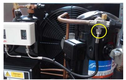
service valve), it should be to a valve with two gauge ports, and it must be connected to the front seat port, as circled in the example valve in the photo.
